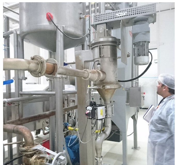
Figure 1. The Self-Cleaning Russell Eco Filter® installed in the peanut processing line at Milhans' production site in Kocaeli, Turkey
