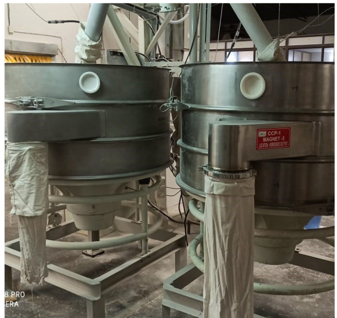
Figure 1. The Finex Ultima™ installed at the Agri Choice Food Products Pvt Ltd plant
