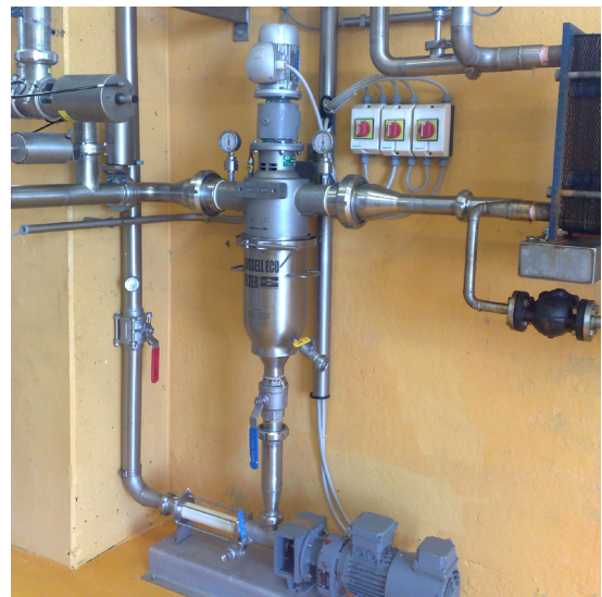
Figure 1. The Self-Cleaning Russell Eco Filter® installed at Consorzio Latterie Virgilio
